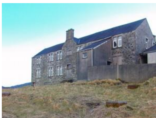
Figure 7. The former Lochmaddy hospital.
