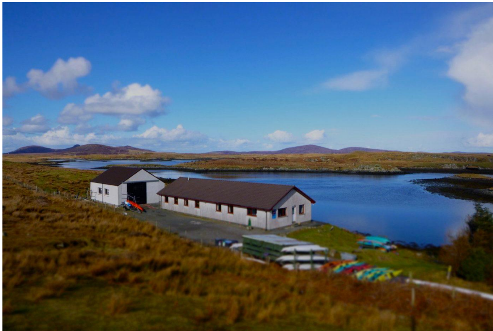
Figure 3. Photograph of former Lochmaddy Outdoor Centre
